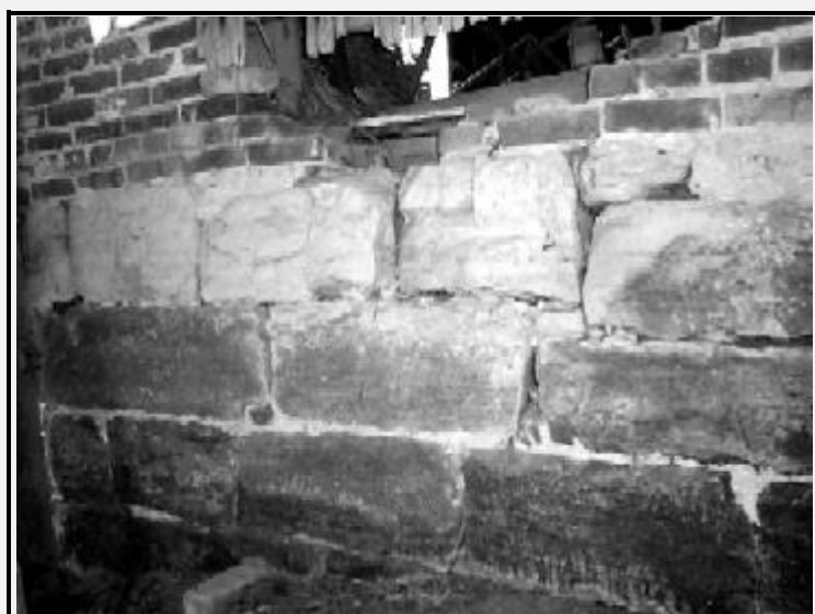
FIGURE 6. FOUNDATION NEAR BACK LEFT CORNER OF MILL NEAR CREEK BANK.
